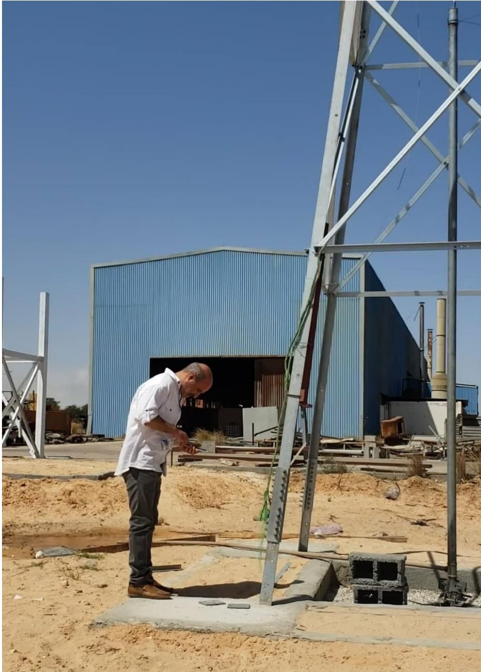
Figure 3-68. Rotor and tower installation.
