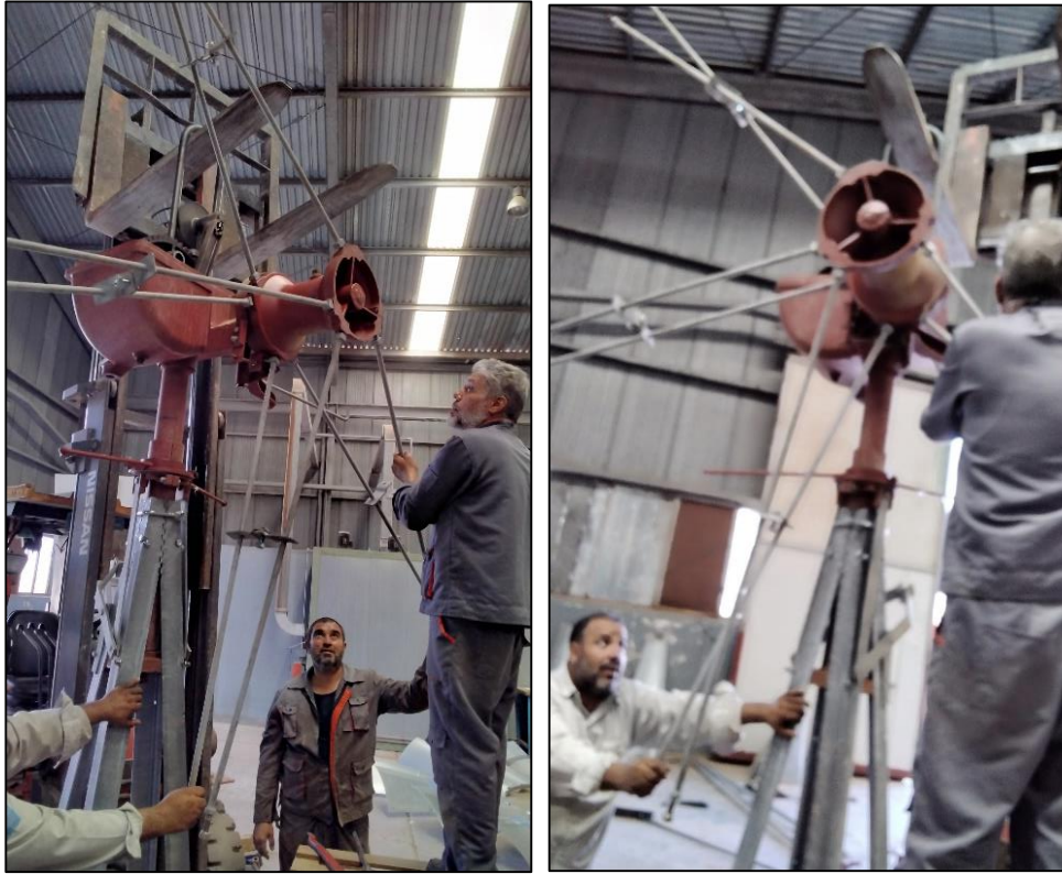
Figure 3-64. Installing the Rotor Arms into the Hub.
