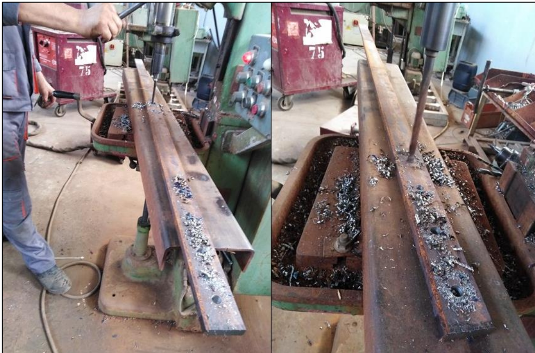
Figure 3-58. Drilling passing holes of the Outer Rotor Bands.
