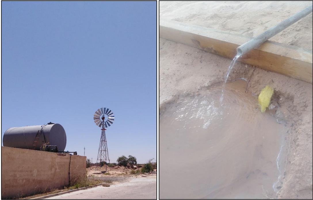
Figure 3-69.Extracting water from the well by the windmill system.
