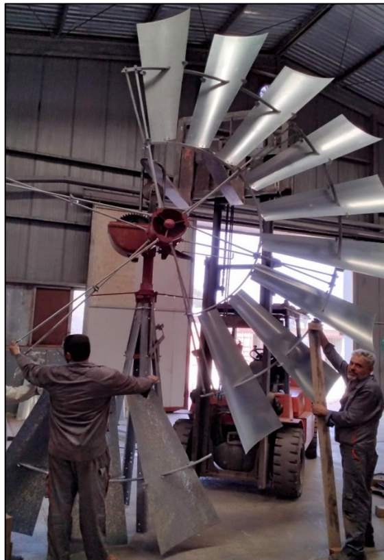
Figure 3-65. Installing the 4th Sails section.
