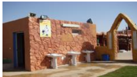
Fig.7 Toilet rooms, in the Sixty's Rest House, source, the researcher (2010)
